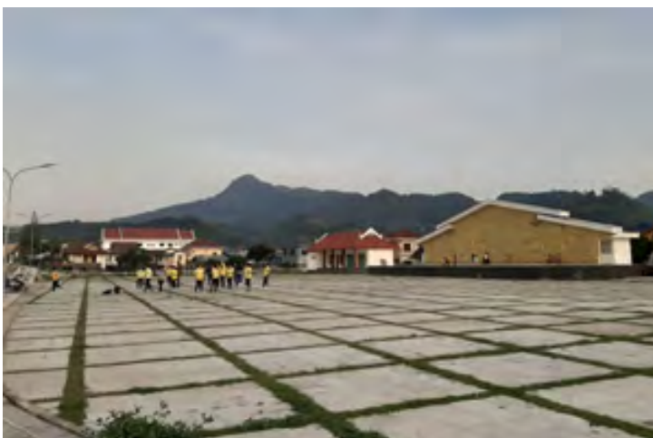
Figure 99. Examples of existing infiltration areas in Sam Neua town Source: (PUW, 2019)
