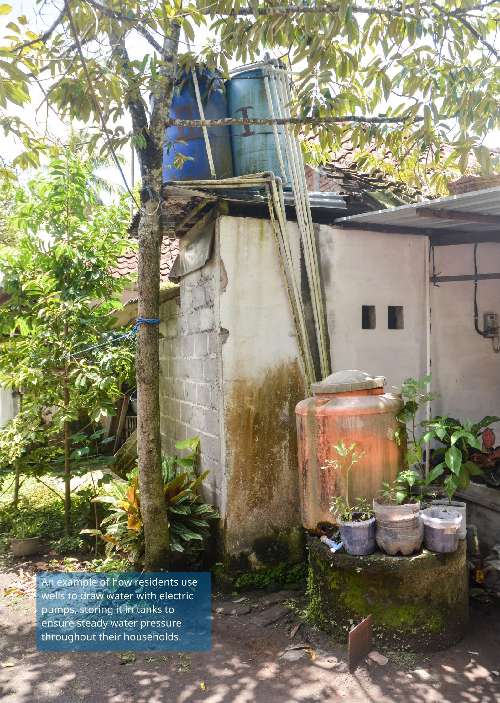
An example of how residents use wells to draw water with electric pumps, storing it in tanks to ensure steady water pressure throughout their households.
