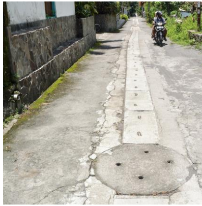
(b) Drainage Channel in the Middle of the Road
