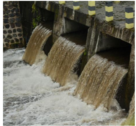
(c) Boyong River used as Primary Drainage System in Rejodani
