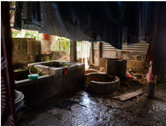
Figure 3.14. Synthetic wastewater from Batik Industry Source: PolyUrbanWaters Team, 2024
