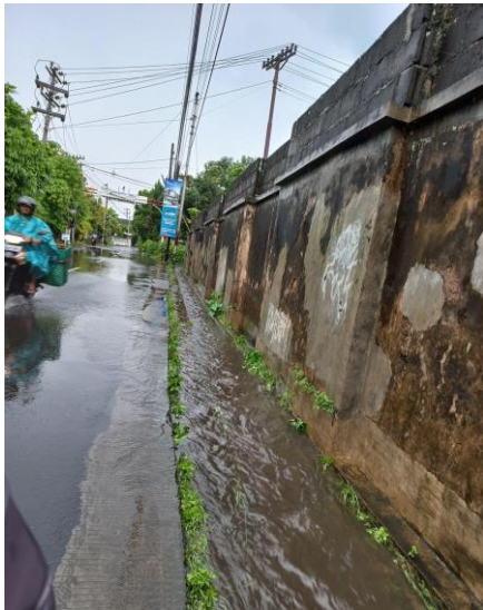
Figure 3.23. Overflowing Drainage in Local Road – Unbalanced built environment and conservation area could decrease the catchment function as natural recharge area and increase the surface runoff Source: Field Observation, 2023
