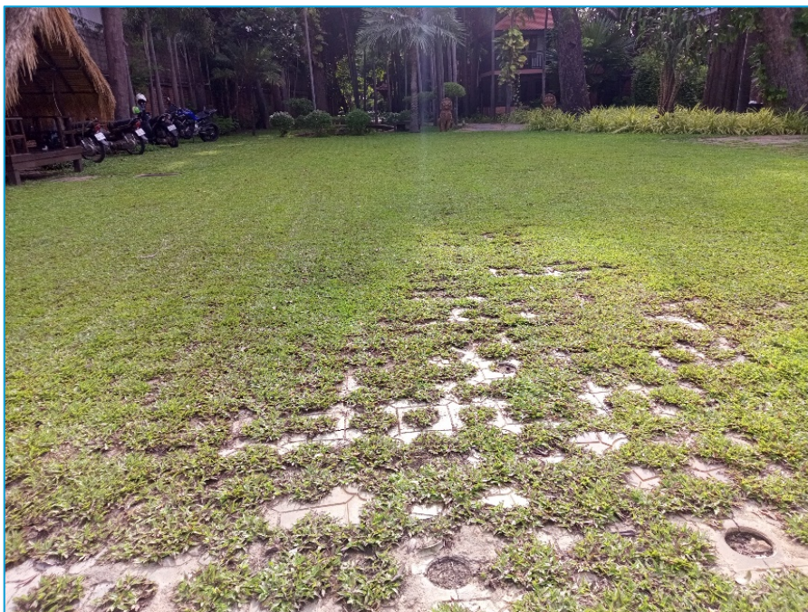
Figure 17: Example of permeable concrete surface used for parking on private property in Krong Siem Reap, Cambodia (Source: Own Photo taken in 2024)
