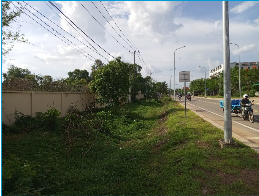
Figure 16. An example of a ditch between main road and property wall in Krong Siem Reap that can be redesigned to act as a bioswale (Source: Own photo take in 2024)
