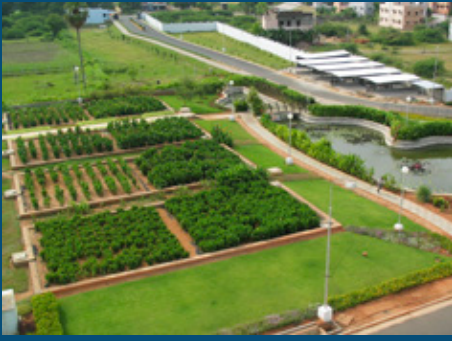
DEWATS system planted filter at Aravind Eye Hospital (Source: BORDA-India, 2015)
