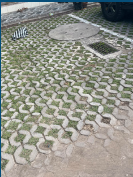
Infiltration stones in settlement area of Sariharjo (Source: PUW & Partners Own Work, 2022)
