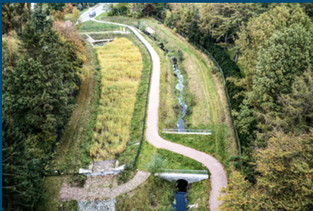
Water retention filter, peri-Urban Area, Hamburg (Source: Hamburg Wasser, 2024)
