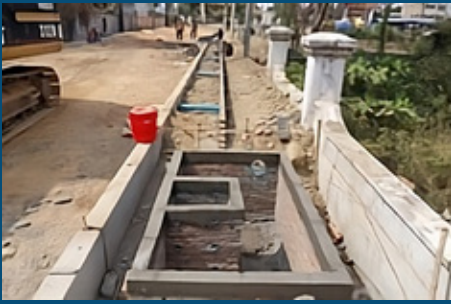
Construction of improved drainage system (Source: BORDA Cambodia)
