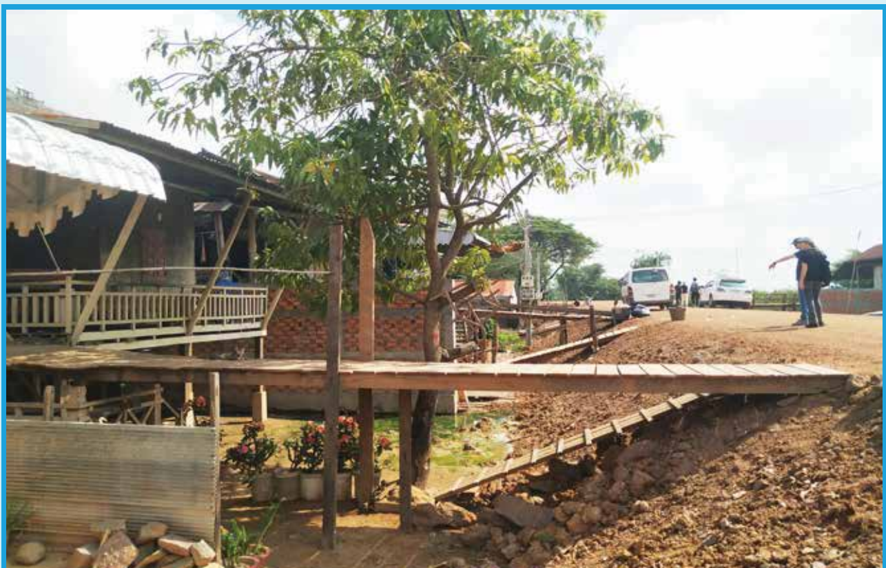
Figure 52 Elevated dirt road in central residential area (Source: Own Photo taken in 2022)
