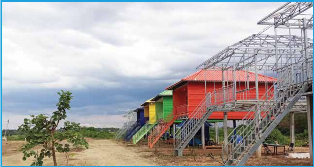
Figure 77 Valuing the lake area for tourism development: Eco-lodges under construction
