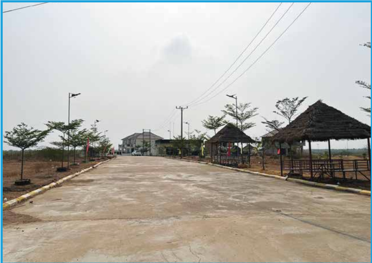
Figure 41 Example of extension towards the lake area (Source: Own Photo taken in 2022)
