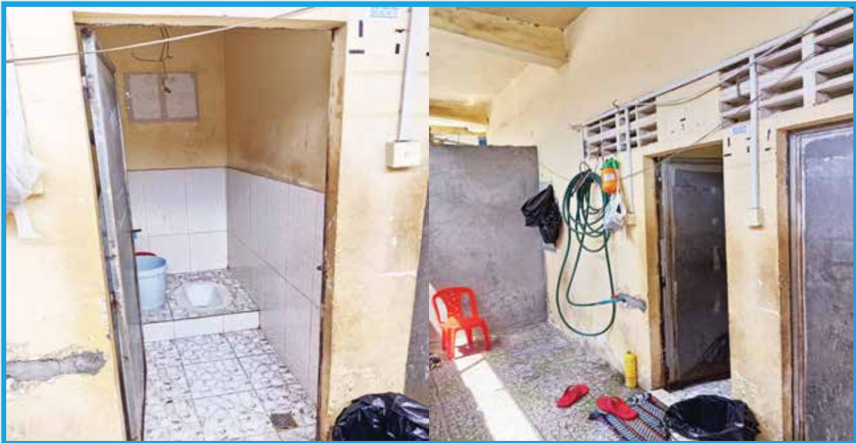
Figure 66 Krong Kratié's Central Bus Station Public Toilets (Source: Own Photo taken in 2022)
