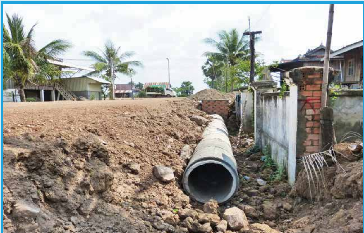
Figure 50 New roadside drainpipe in central residential area (Source: Own Photo taken in 2019)
