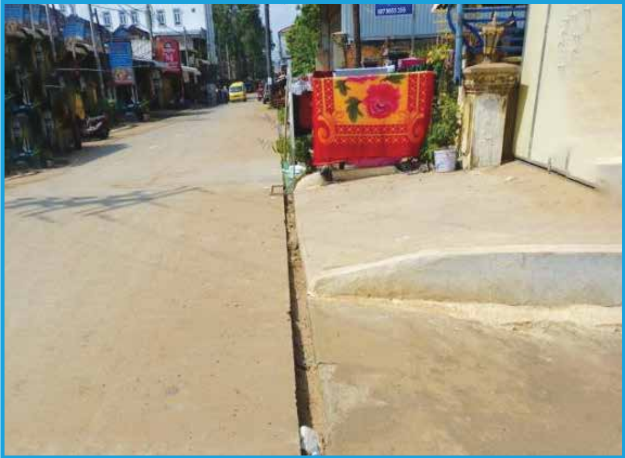
Figure 49 Gutter in central area (Source: Own Photo taken in 2019)
