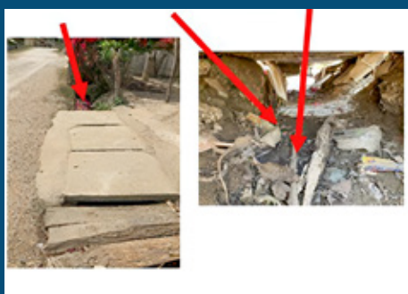
Blocked drainage close to SOS School (Source: Foelster, 2024a)
