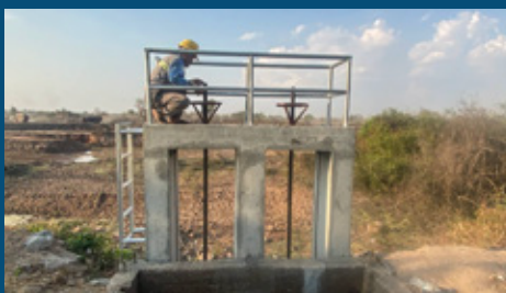
Rehabilitation of existing flood gates in the wetland area of Kratié (Source: PUW & Partners Own Work, 2024)
